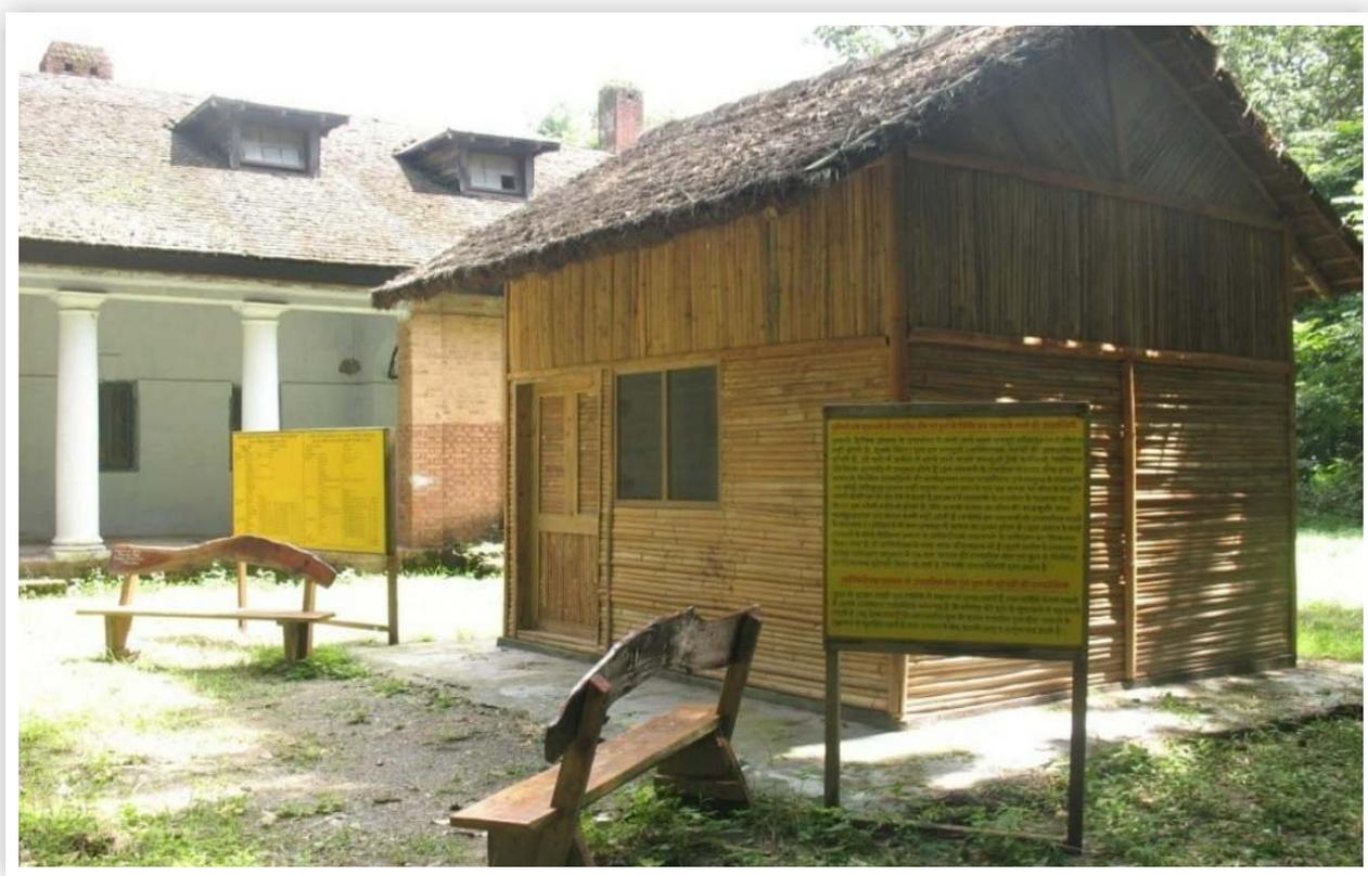
Demonstration structure made of ZiBOC treated bamboo and thatch 2008
